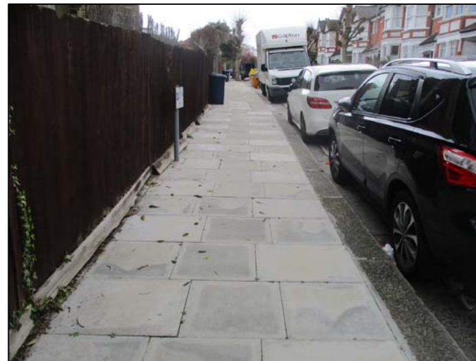
CASE STUDY: NETHERFIELD ROAD, N12
